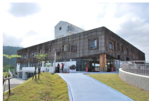
Figure 7. Siao-Lin Elementary School
