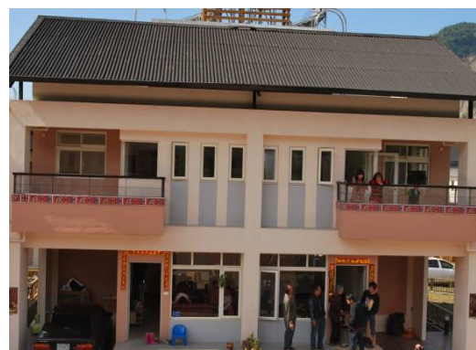
Figure 2. House in First Siao-Lin Village
